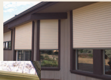
Exterior rolling shutters
